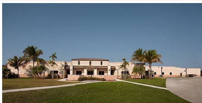
PROJECTS: HOMESTEAD AIR FORCE BASE - BLDG 191
