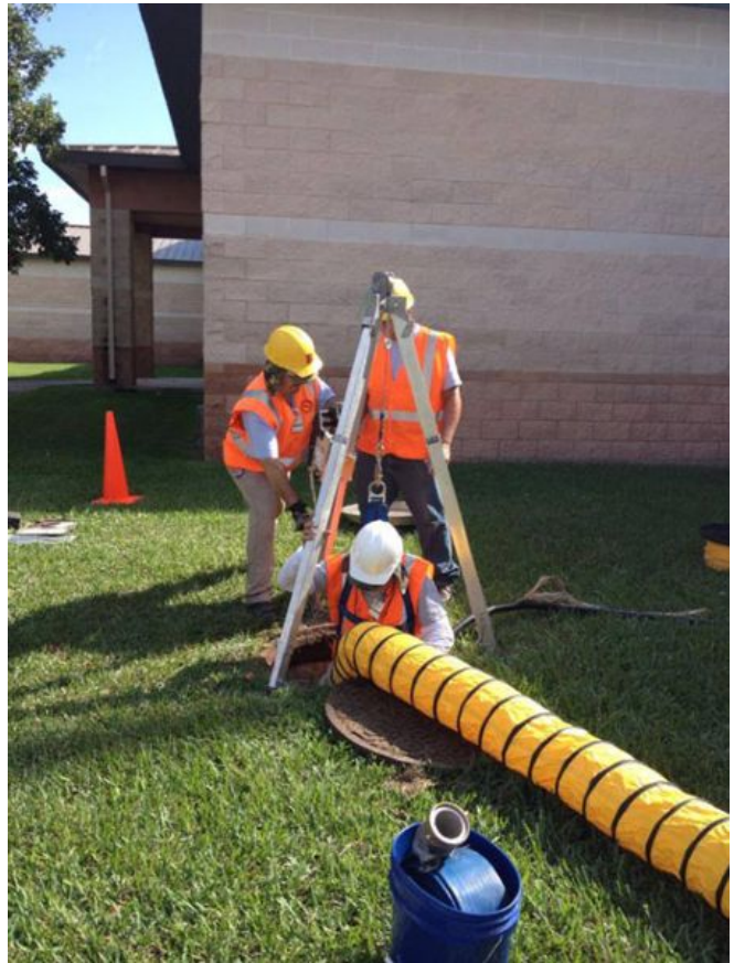
Services: Underground Work
